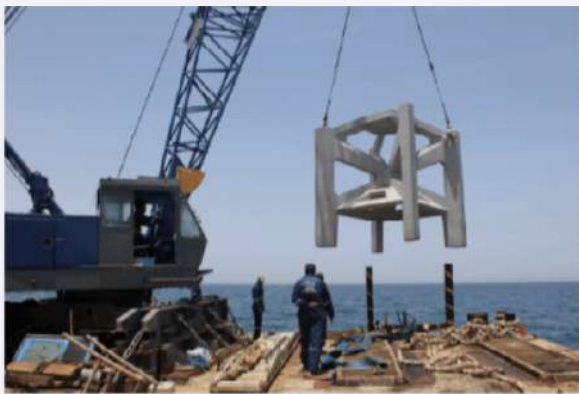
Figure 1. Dismantling of Fish Cube module
