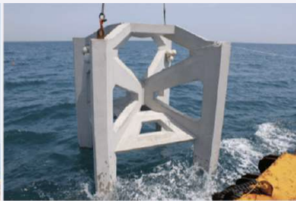
Figure 2. Lowering down the module on the seabed
